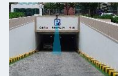
Underground parking lots
